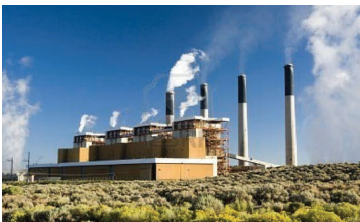
Coal Electrical Generation
