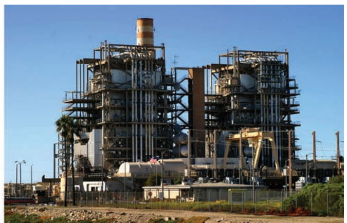
Natural Gas Electrical Generation
