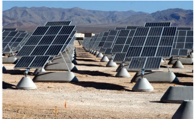
Solar Electrical Generation
