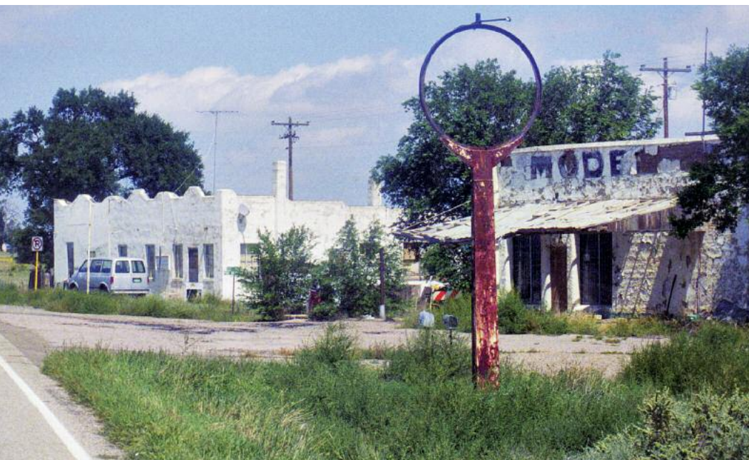
The little town of Model is truly abandoned. Doors sag in their frames, and the rim of an old fuel sign dangles from its painted pole, but gnarling fingers of thorny weeds have not yet overcome the gravel of old streets.
